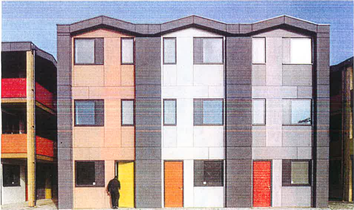
Y Cube 'move on' housing in Merton, London.
